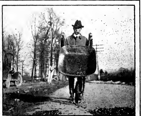
USING THE NEW WHEELBARROW TYPE ROAD REPAIR MATERIAL HEATER
